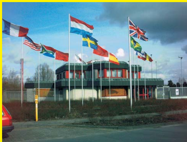
Entrance to the Uranium Enrichment Plant Gronau credits: Falk Beyer
