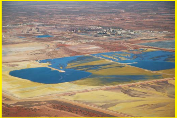
Tailing ponds at the Olympic Dam Mine in Australia credits: http://nukingtheclimate.com
